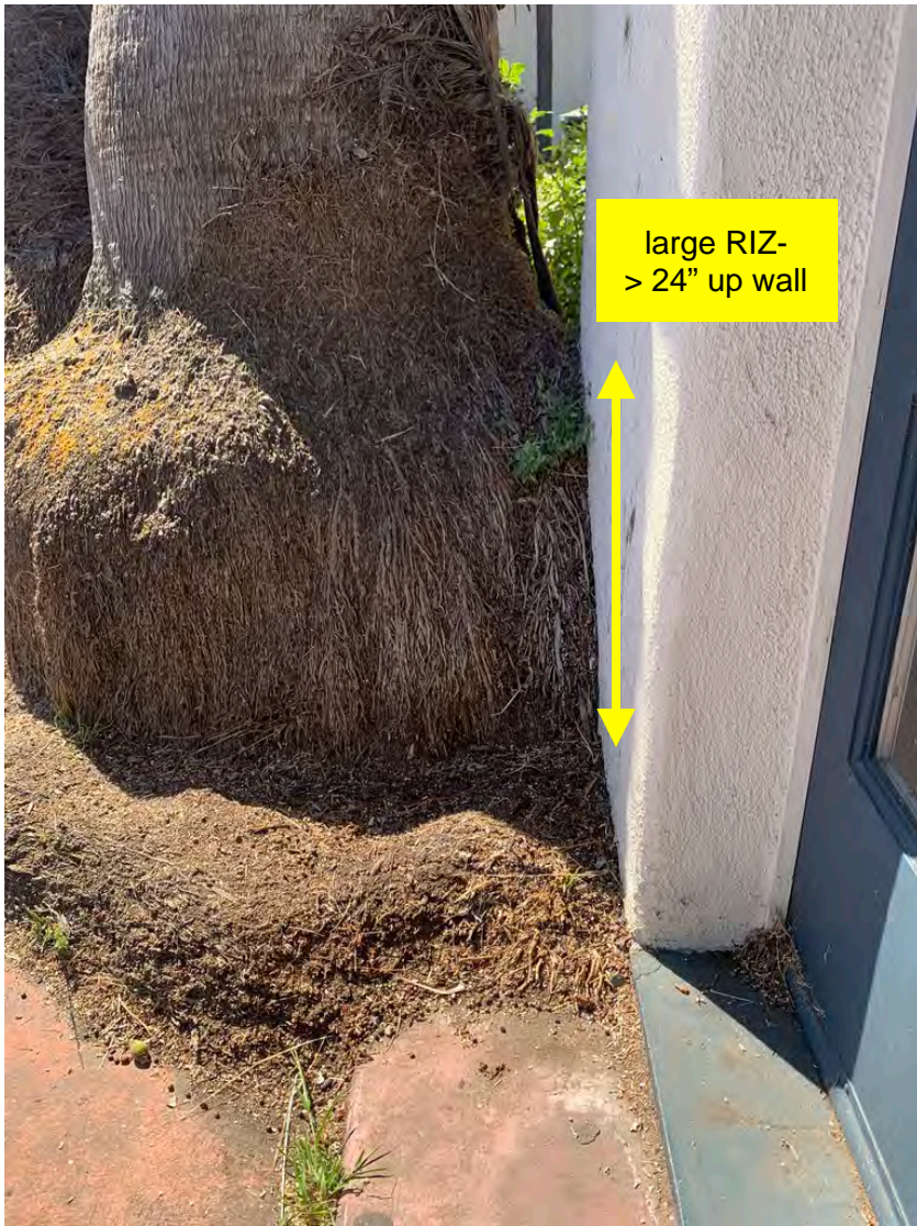
Above left: extended RIZ pushing wall and blocking drainage.
